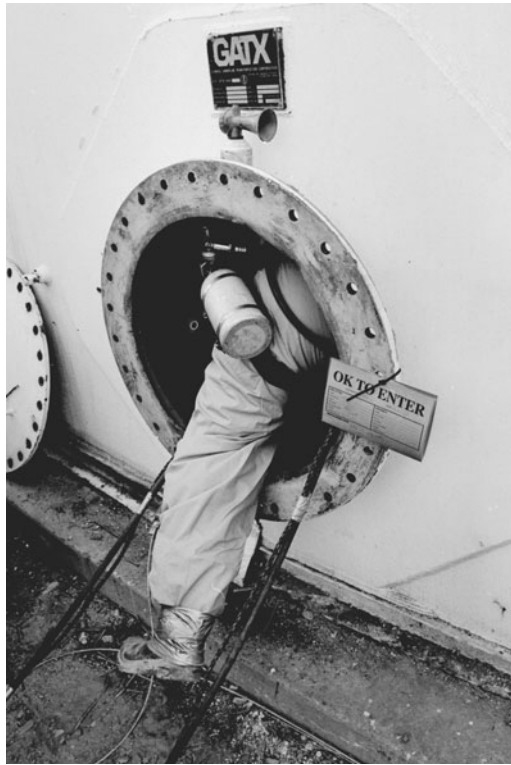
Figure 12.1 Confined spaces are enclosed locations, such as tanks, sealed rooms, reaction vessels, and pipelines. They are also created when processes are contained, which is one form of engineering control to prevent exposure, but sometimes have to be entered for maintenance or repair. They are especially hazardous because entry and exit may be difficult in an emergency, the air may be contaminated, fumes may build up to create a fire or explosion hazard, and oxygen levels may be too low to support life. This worker is entering a tank to repair damage after an earthquake in California. He is carrying self-contained breathing apparatus (SCBA, the metal tank visible next to his leg), which is a supplied air respiratory personal protection device providing about 25 minutes of air, enough time to escape in an emergency. The tank has been checked carefully for oxygen level and to ensure that there are no toxic or flammable gases present, as shown by the permit tied to the flange (an example of administrative controls ). Workers who enter confined spaces are required to work with a coworker (a “buddy,” not seen in the photograph) who stays outside and carefully monitors the situation and who will call for help in case of emergency, another example of administrative controls . Note that the worker’s boots are taped to his pants in order to keep dust and chemicals out, another example of personal protection . (Photograph by © Earl Dotter, all rights reserved.)
