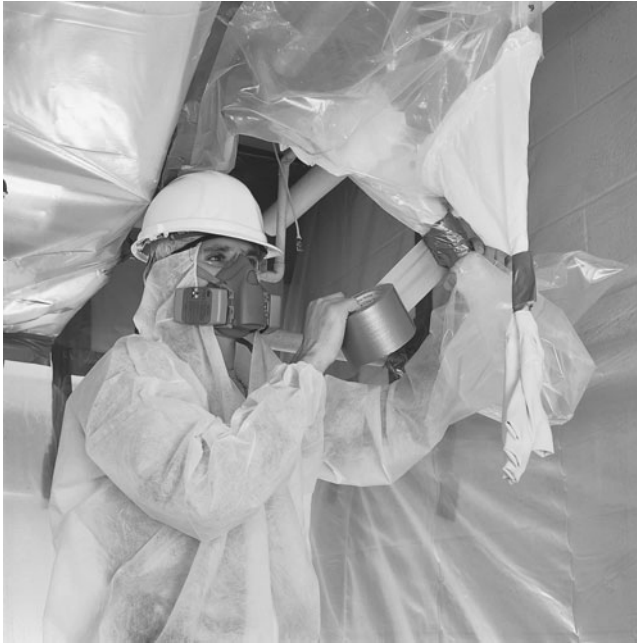
Figure 12.3 This half-face mask respirator is an example of an air purifying device. The cartridges on either side of the mask contain different filters or absorbing agents and are chosen for the specific hazard. The worker using the respirator is preparing a workplace for asbestos abatement by sealing it off with plastic sheeting, and he is also wearing protective clothing, safety glasses, and a hard hat. (Photograph courtesy of the manufacturer, © 3M Corporation, all rights reserved.)
