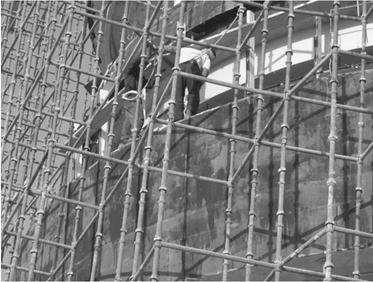
Figure 6.6 This worker is working on open scaffolding without a hardhat but is using basic fall protection (see the rope leading under his T-shirt). (Photograph by Seifeddin Ballal, King Faisal University, Saudi Arabia.)
