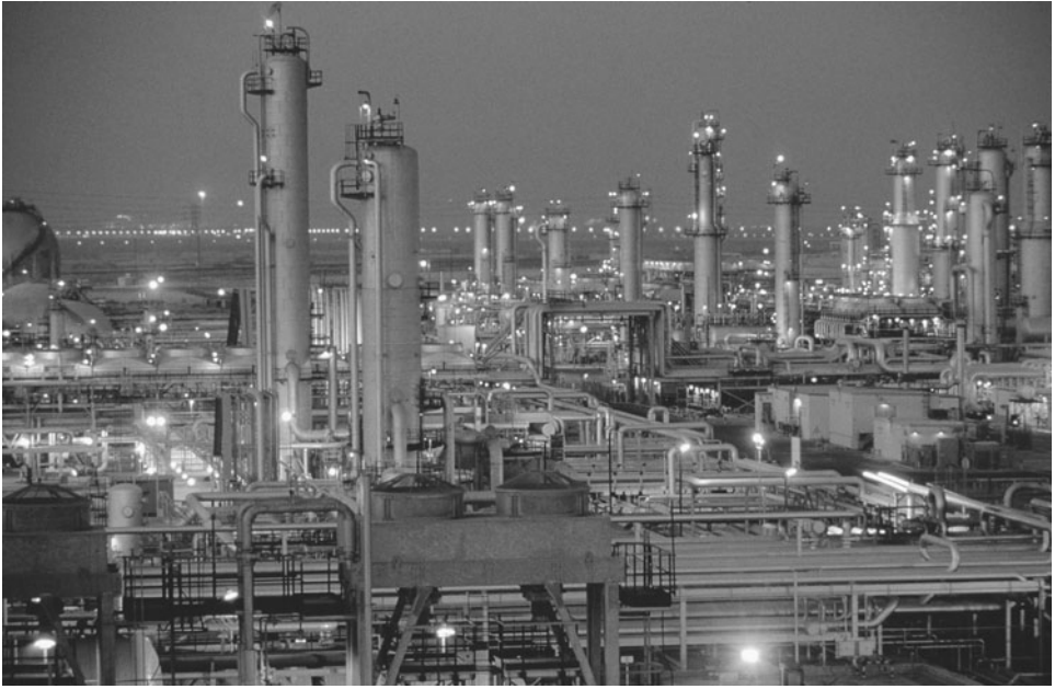
Figure 19.4 The oil refinery in Ras Tanura, Saudi Arabia, is one of the largest in the world. Refineries are basically elaborate plants for distillation of petroleum into lighter fractions, such as gasoline, and heavier fractions, such as kerosene, which are then sold or shipped as different products. Occupational health management has to be strict in a refinery because of hazards involving safety, fire, and toxic chemicals. (Photograph courtesy of Saudi Aramco World, SAWDIA.)
