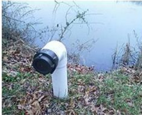
Gambar 4.4 Hydrant Barel-Kering
