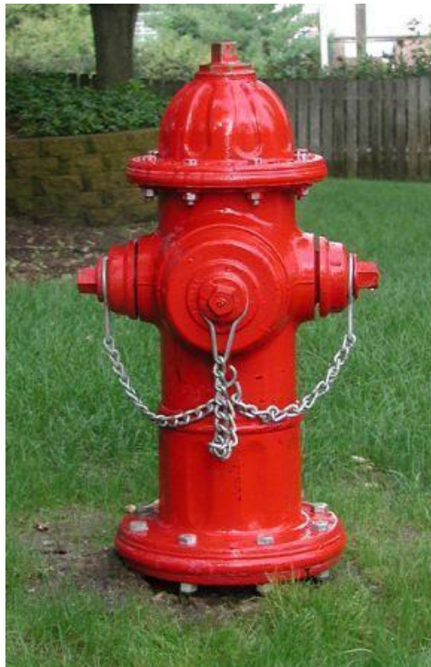
Gambar 4.3 Hydrant Barel-Basah
